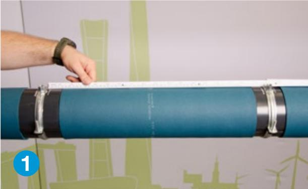
Measure the length of the straight pipe between both ArmaFix metal clamps.
