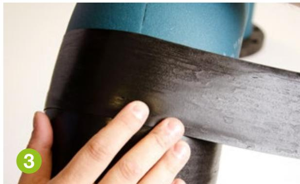
Apply moderate tension to the self-welding covering material as you wrap it around the pipe. This helps ensure a secure and uniform application.
