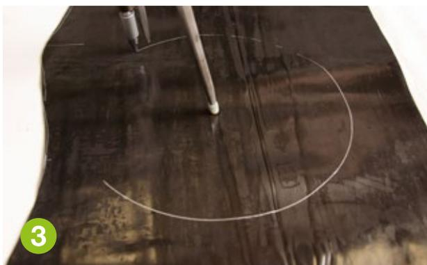
Cut the end cap disc with the radius of the insulated pipe and add an extra 20mm.
