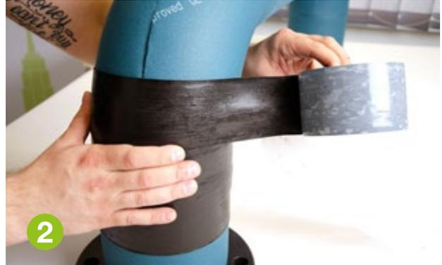
Wrap the self-welding covering material around the insulated pipe, ensuring that each new layer overlaps the previous one by a minimum 20mm.
