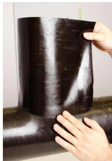
Apply our Arma-Chek Wrap product with an overlap of 20mm onto the body.
