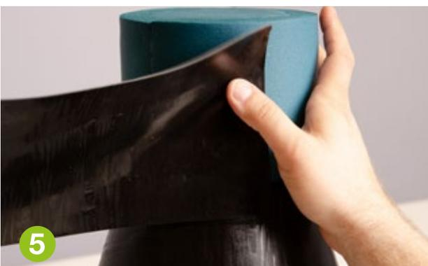
Apply our Arma-Chek Wrap product with an overlap of 20mm onto the body.
