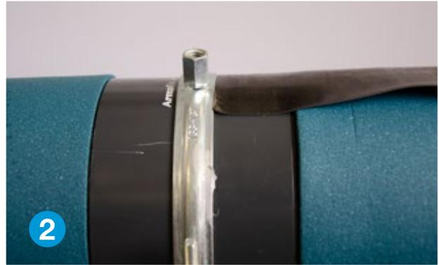
Apply our Arma-Chek Wrap product onto the surface of the ArmaFlex insulation and on the ArmaFix pipe hangers.
