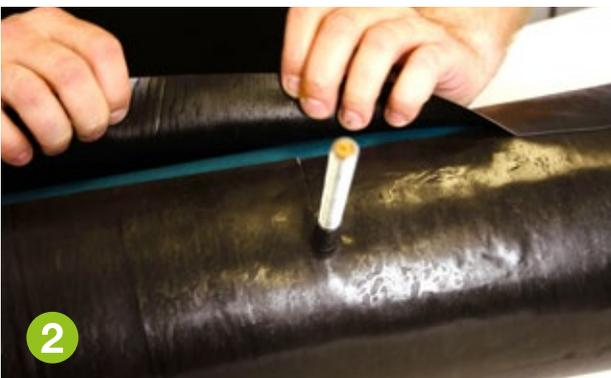
Proceed as a straight pipe covering. Include a cut-out with a diameter equal to the rod diameter.
