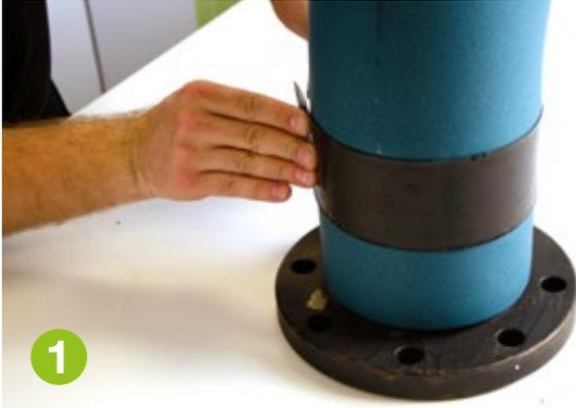
If the diameter of the bend is  $>90\text{mm}$ , the wrapping method can be applied. Use our Arma-Chek Wrap product with 70mm width and begin the wrapping process at one end of the bend and work your way towards the other end.
