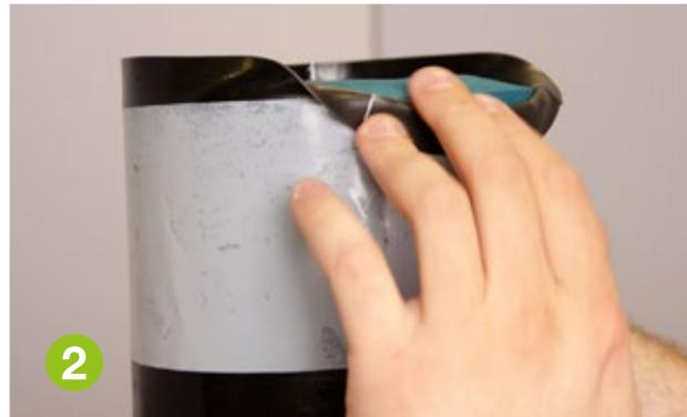
Fold back the longitudinal extra 20mm. To prevent the folded section from sticking to itself, it is essential to insert a release paper between the folded piece and our Arma-Chek Wrap product surface.
