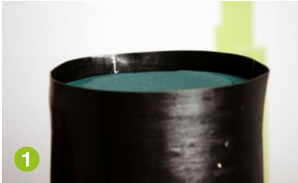
Apply straight pipe insulation as mentioned previously until the end of the pipe. Add an additional 20mm for the overlap.
