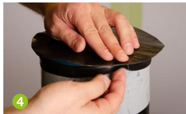
Apply the disc to the end of the pipe and unfold the first applied covering. During the vulcanisation process, it is important to match the edges of the end cap and pipe covering.
