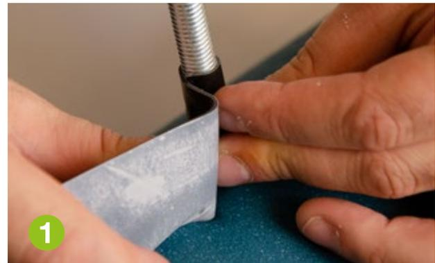
Apply a small piece of our Arma-Chek Wrap product around the rod with a length of 30-50mm.
