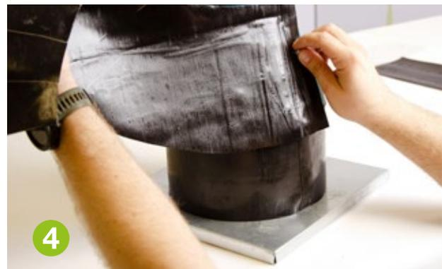
Starting at one end of the pipe reducer, carefully wrap the self-welding material around the pipe. Ensure that the material is tightly secured without gaps.
