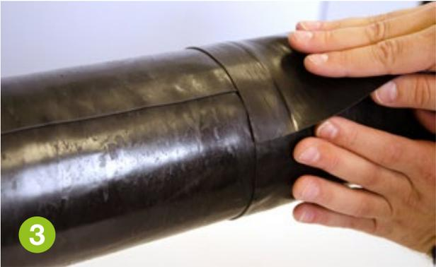
Always stagger the longitudinal overlaps and position them to the side with the seams downward facing to provide watershed.
