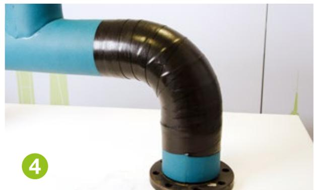
Repeat the wrapping process, maintaining the overlap and tension, until you reach the opposite end of the bend.
