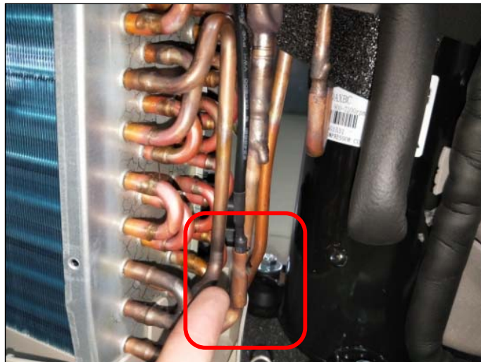
⑤Condenser temperature sensor
