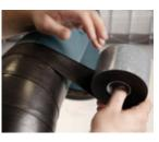
around the insulated pipe with an overlap of 20 mm. The self-welding material
